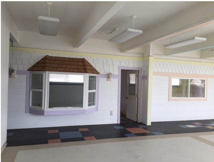
Enclosed rooms adjoining the open area.
