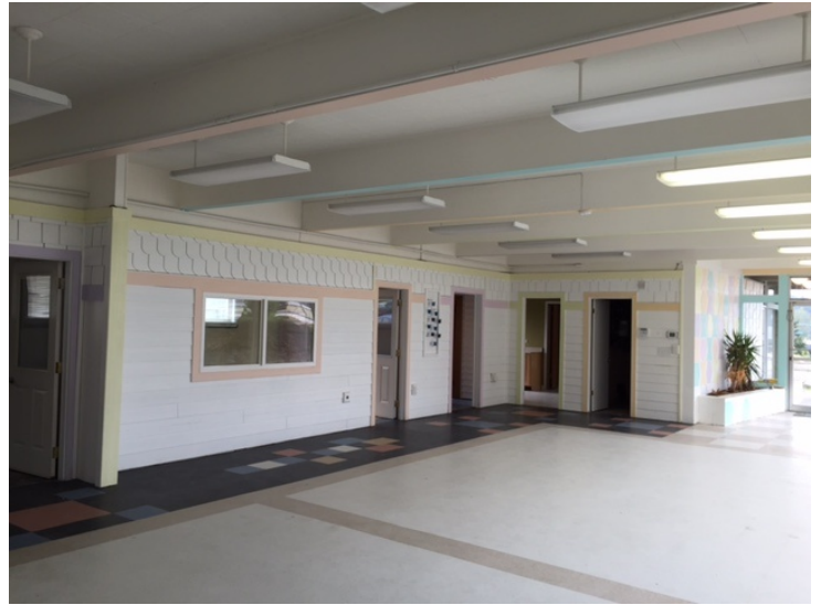
Interior view toward the entry and enclosed rooms.
